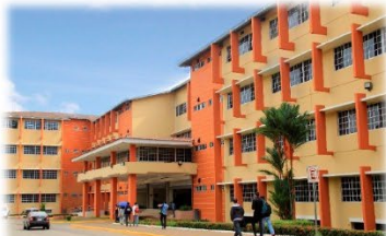
Building # 1: Civil, Industrial, Electrical and Mechanical Schools
